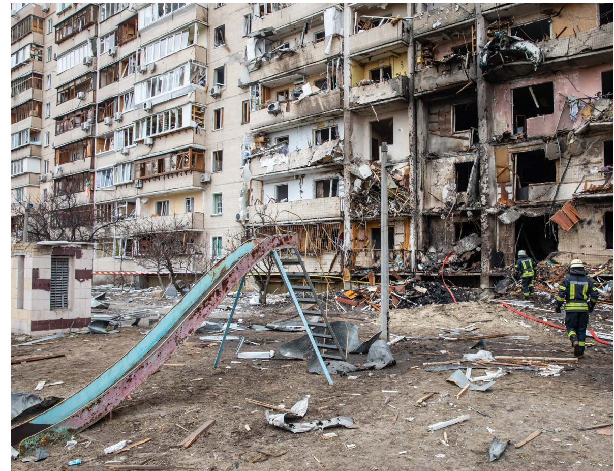
Damaged by enemy aircraft: a residential building in Kyiv awaits reconstruction.
