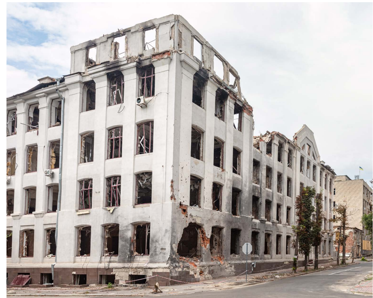
To be rebuilt: a destroyed building in Kharkiv.
