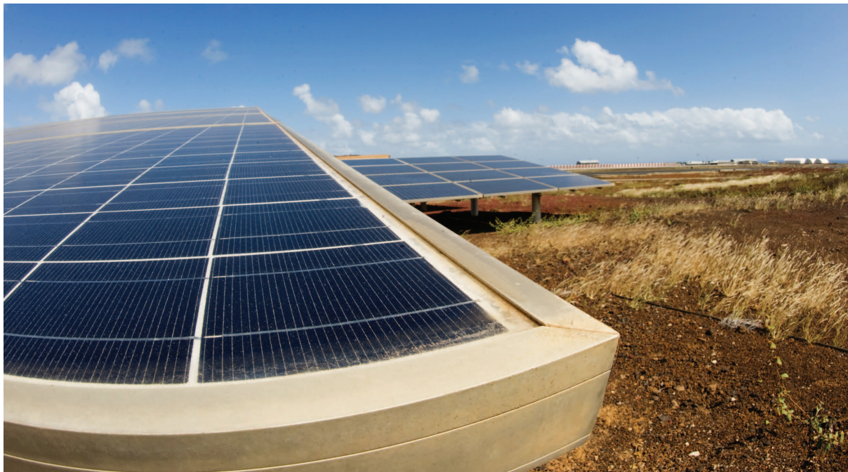
Solar panels are the sole source of energy for the runway lights at the 45th Operations Group, Detachment 2, at Ascension Auxiliary Airfield (AAF), South Atlantic Ocean. (U.S. Air Force photo by Lance Cheung)
